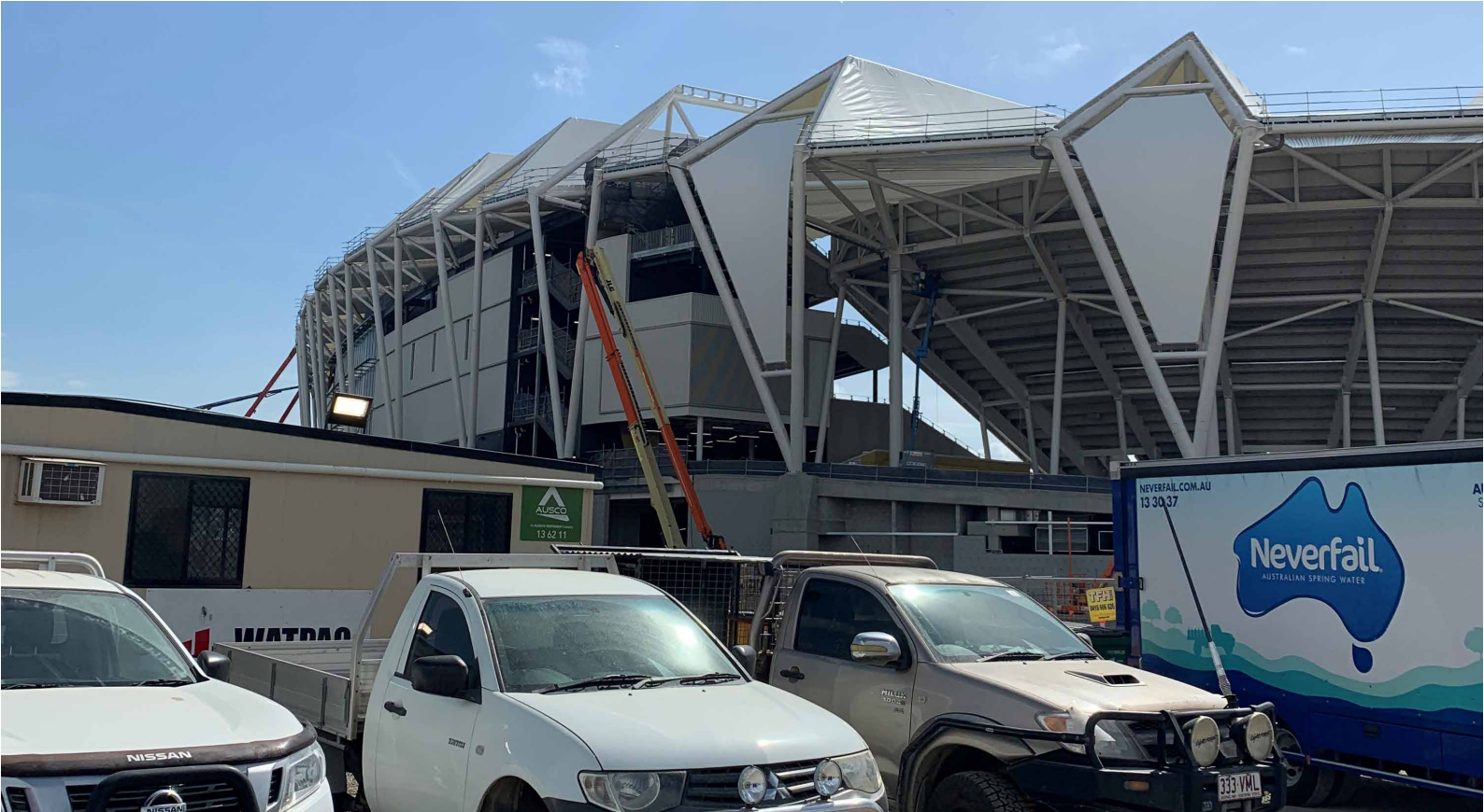
First on site August 2017
